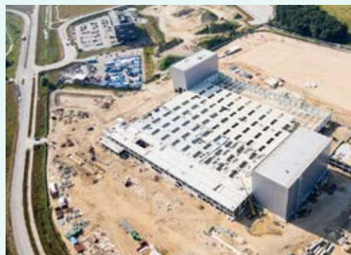
Northvolt Dwa Construction November 2022
