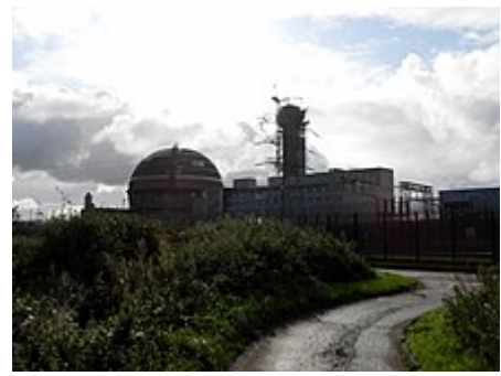
Pile 1 being dismantled in 2018
