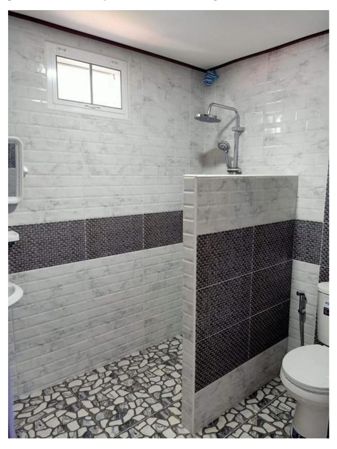
Wall should cover the wall surface with materials that are easy to clean, such as ceramic tiles. Or in case of bare polishing, coat with another layer of polish to prevent moisture accumulating and easier to clean.
