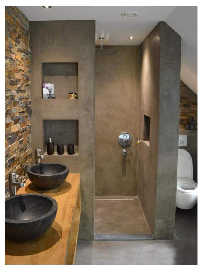
The floor area of the shower may be designed to have a floor level below the dry zone about 5-10 cm to prevent water from flowing out to the floor.
